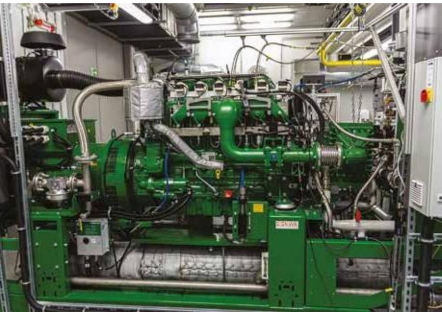
IL COGENERATORE CONVERTITO A IDROGENO PRESSO L'OTH DI AMBERG-WEIDEN, IN GERMANIA
