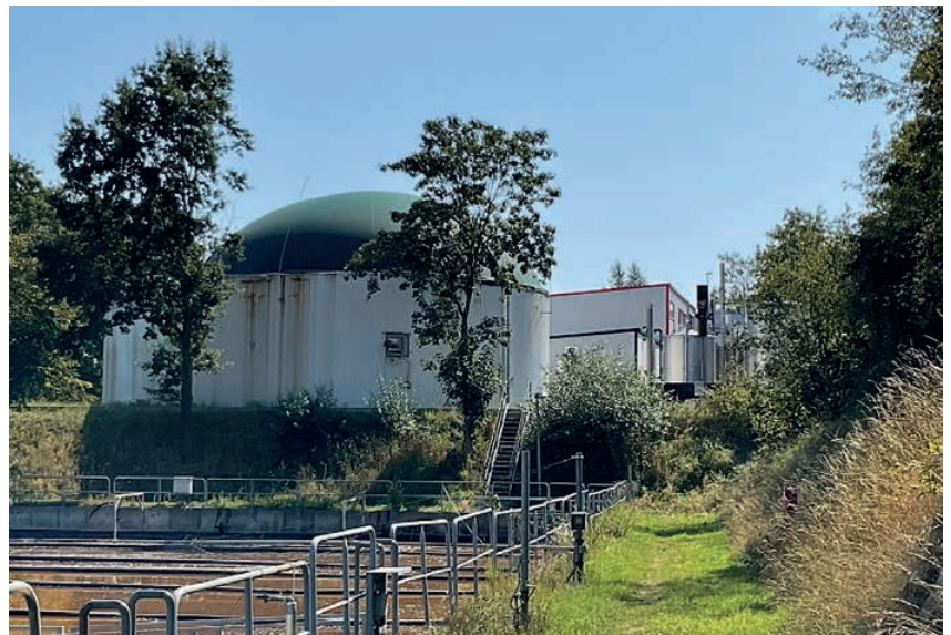
Figure 2. Biogas facility with fermenter
