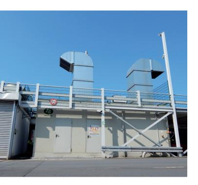
emissions of max. 45 dB (A) at a distance of 10 m), there was an equally impressive solution for the installation's appearance: the concrete sound hood together with the agenitor were inserted into the hospital's parking structure. To do so, a recess was made in the top deck, through which all of the components were lowered in using a crane. The colour of the concrete sound hood was matched to the colour of the parking structure.
