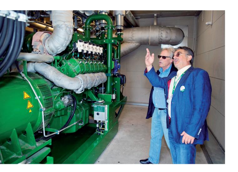
Jühnde is the first bioenergy village of its kind in Germany. Using biomass and two 2G avus 500plus plants (550 kW electrical and 526 kW thermal capacity), amongst other things, the village generates twice as much electricity as it needs – additionally the adjacent houses are very efficiently supplied with heat.
