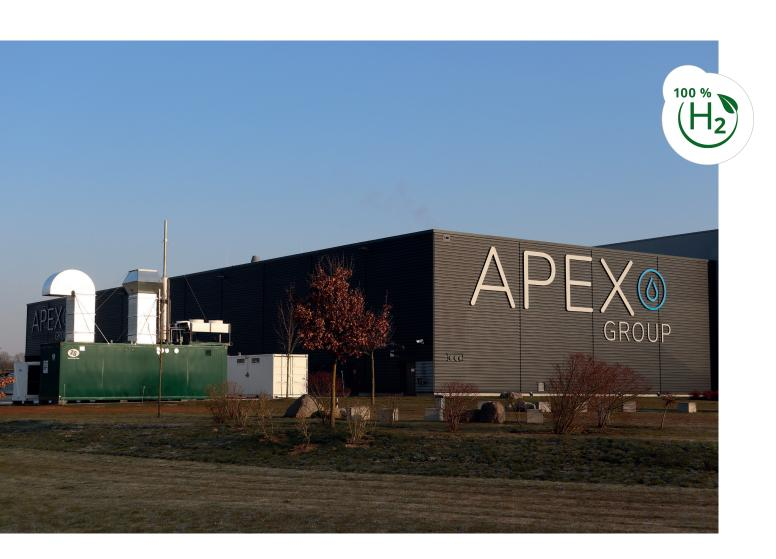
At APEX Energy Teterow GmbH in Rostock-Laage, Germany, an agenitor 404c  $H_2$  from 2G Energy with an electrical output of 115 kW (129 kW thermal) was commissioned in April 2020 as a plug-and-play container solution. According to the industrial requirements of APEX, the CHP system serves for self-sufficiency.
