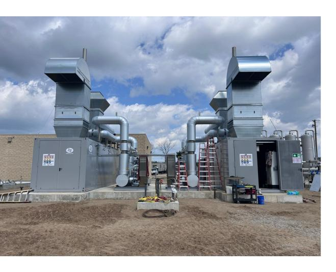
The Clinton River Water Resource Recovery Facility in Michigan, USA, is a municipal facility that focuses on wastewater treatment. With the aim of reducing operating costs while making efficient use of sustainable energy sources, the wastewater treatment plant opted for a modern CHP solution from 2G Energy. The generation of electricity and heat from existing sewage gas contributes significantly to the optimization of the onsite energy supply.
