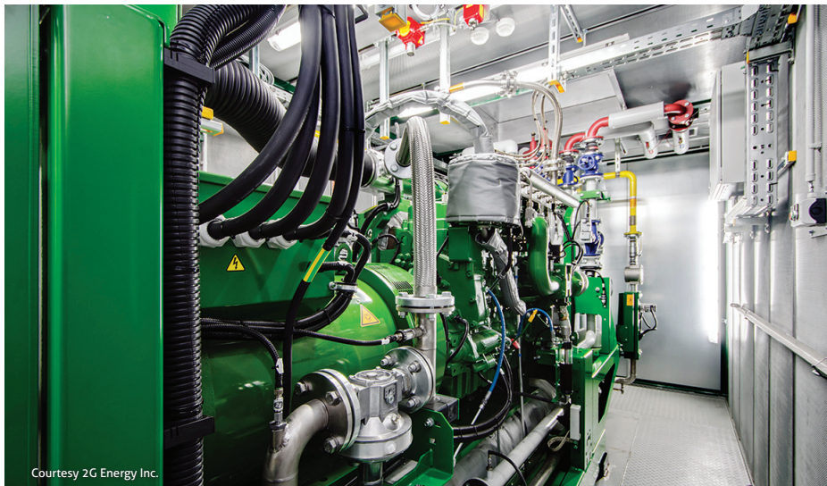
Hydrogen-ready CHP technology at Kirkwall Airport, Scotland.
