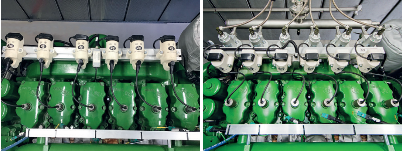
Each natural-gas driven 2G CHP (l.) can be retrofitted for the use with hydrogen in the future (r.)
