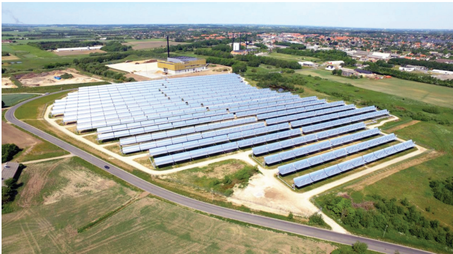
4. Danish utility Brønderslev Forsyning in 2018 replaced seven gas-fired CHP units and began operating a district heating plant that utilizes two wood chip boilers, heat pumps, and solar heating from a 27,000-square-meter parabolic trough concentrated solar power plant supplied by Denmark's Aalborg CSP. The boilers and solar heat supply energy to a Turboden Organic Rankine Cycle (ORC) turbine. During the summer months, the wood chip boilers can be shut down and the solar collectors take over heat production. The ORC system converts 20 MWth into 4 MWe and 15 MWth. Courtesy: Brønderslev Forsyning
