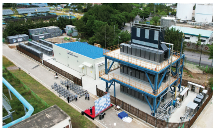
2. Public power generator Korea East-West Power's (EWP's) 4.2-MW CHP plant featuring Bloom Energy solid oxide fuel cells (SOFCs) opened in June 2022 in Donghae City, South Korea. The utility uses heat from the plant to supply hot water to a swimming pool at the adjacent Bukpyeong Leisure Sports Center. SK Ecoplant developed a custom heat recovery system for the project. Courtesy: SK Eco-plant.
